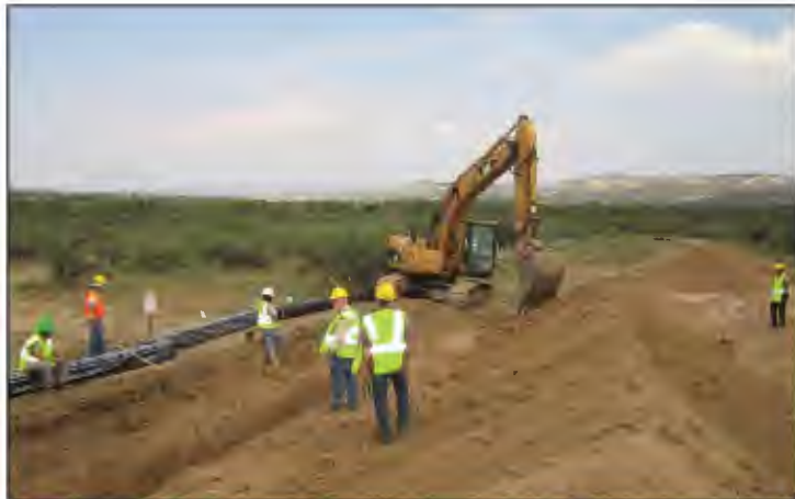
Homestead utility work begins with VVAC crews monitoring the excavation for any archaeological indications.
