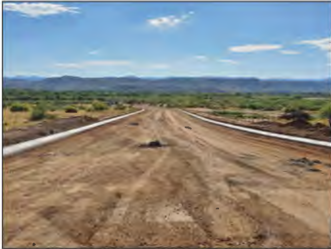
Homestead Parkway curbs
