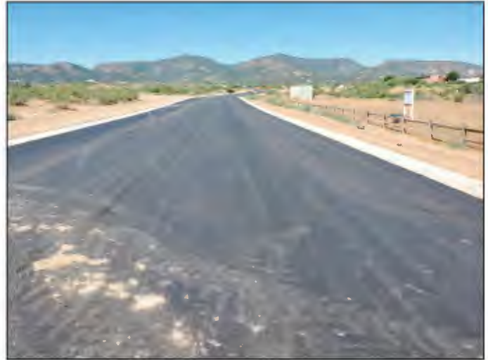
Homestead Parkway completed
